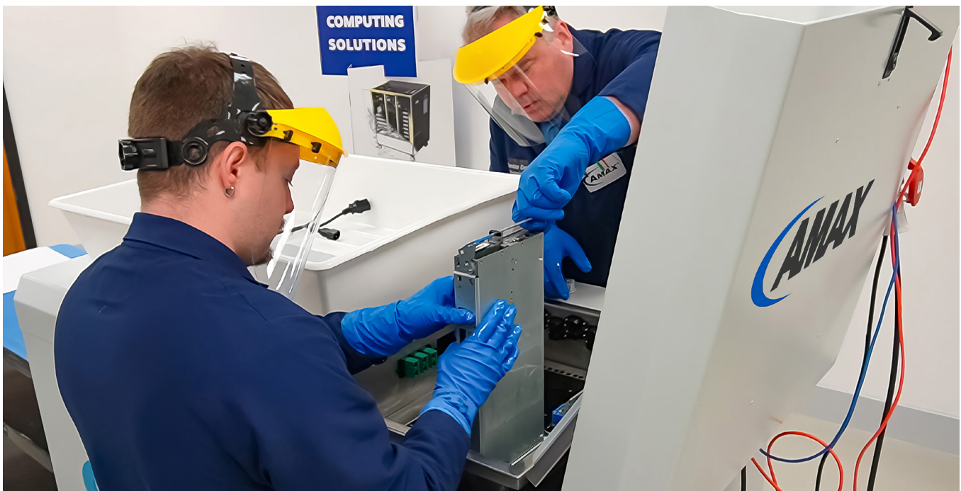
AMAX engineers working on an immersion cooling solution
